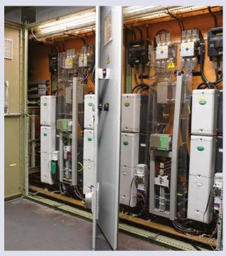
Three of three massive aluminium extrusion presses, at Alcoa in Hannover, now depend on iMEC variable speed drives and, as well as dramatically increasing production time availability, increasing throughput by 10% and decreasing maintenance costs, the installations have cut energy consumption by a huge 40%, saving thousands of kilowatt hours of energy every year!
