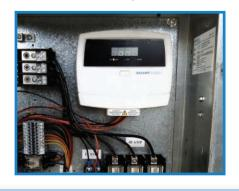
The ECO³™ units were installed to optimize the compressors in the air conditioning systems. Smartcool installed amperage and temperature loggers in order to monitor the performance of the equipment. This information was collected as the ECO³™ units were switched between OFF and ON modes to gain a comparison of performance with and without Smartcool technology. The energy savings shown here were achieved with no discernible impact on temperature.
