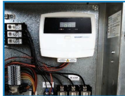
The ECO<sup>3</sup>™ units were installed to optimize the compressors in the air conditioning systems. Smartcool installed amperage and temperature loggers in order to monitor the performance of the equipment. This information was collected as the ECO<sup>3</sup>™ units were switched between OFF and ON modes to gain a comparison of performance with and without Smartcool technology. The energy savings shown here were achieved with no discernible impact on temperature.
