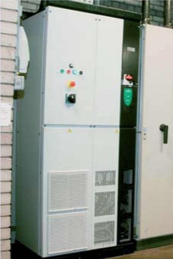
The installation of a large free-standing iMEC variable speed AC drive has improved temperature control in a food company's chilled rooms, and is well on the way to delivering a massive saving of around £23,400 in their annual electricity bill – a cut of 50% of the plant's total power usage!
